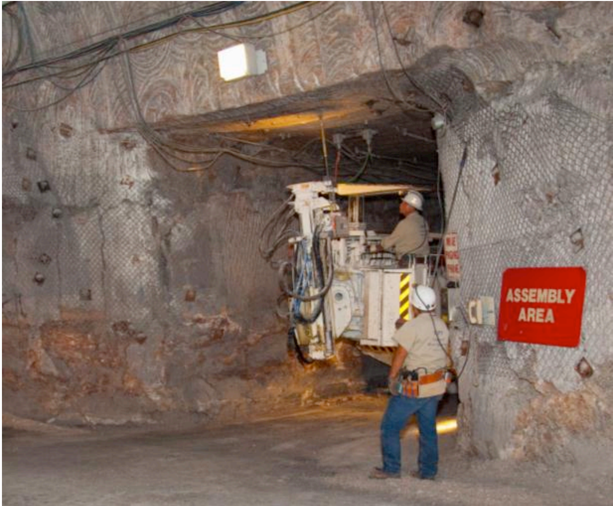
Mining personnel install a rock bolt that helps stabilize the rock formation in the WIPP underground facility.
